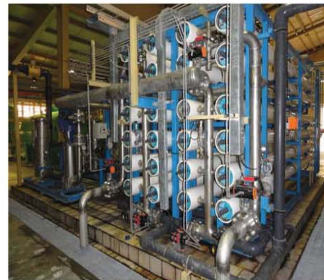
YAZD Thermo-Solar Power Plant Water Treatment Plant(R.O., Demin., Regeneration System)
