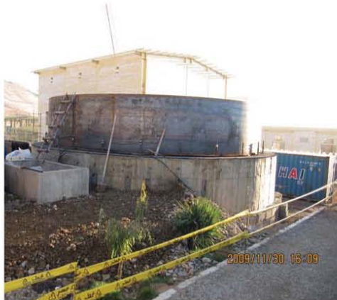
SANANDAJ Combined Cycle Power Plant Demin. Water and Condensate Storage Tanks
