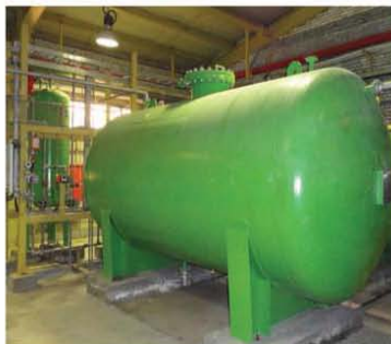
YAZD Thermo-Solar Power Plant Water Treatment Plant(R.O., Demin., Regeneration System)
