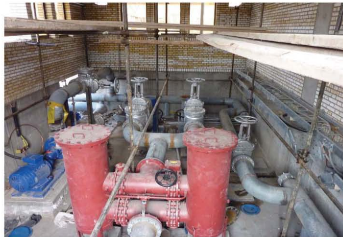
FARS Gas Power Plant-Fuel Oil Unloading & Forwarding Pump House and Piping
