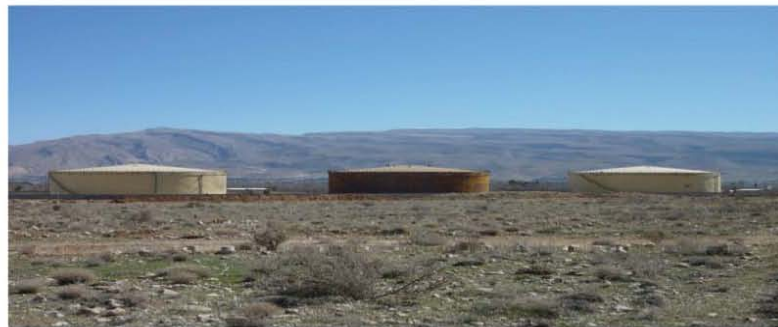
FARS Gas Power Plant- 3 x 20,000 m 3 Fuel Oil Storage Tanks
