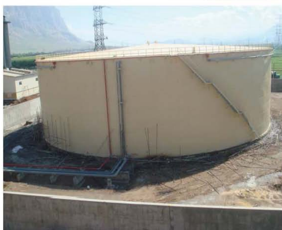
KERMANSHAH GAS POWER PLANT-3 X 33,000 m3 Fuel Oil Storage Tanks
